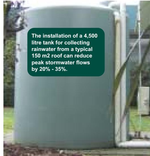
The installation of a 4,500 litre tank for collecting rainwater from a typical 150 m<sup>2</sup> roof can reduce peak stormwater flows by 20% - 35%.
