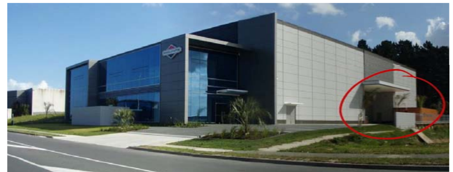
Servicing and storage of containers is located inconspicuously to the side of the building with all effort directed towards focusing attention to the building frontage.
