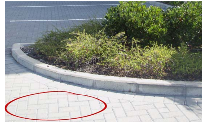
Semi-permeable pavers help to manage storm water issues and can add visual interest to an industrial site.
