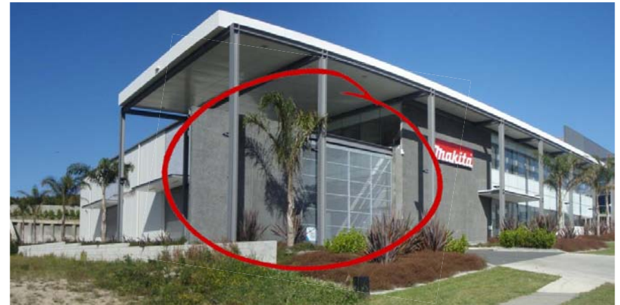
A false façade and gate provides for very secure, safe, and screened servicing, loading/unloading, and storage/collection of wastes away from the street.
