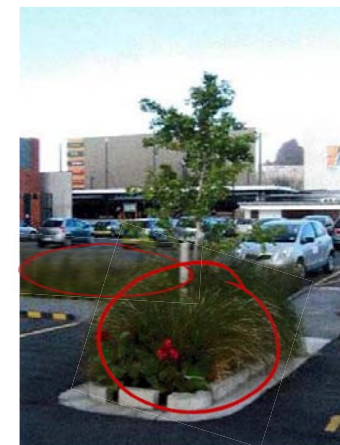
A small raingarden and swale located between parking bays. Source: NorSGA Low Impact Design Code of Practice
