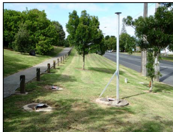
The presence of landfill gasses in these manholes is a Health and Safety risk. To manage the risk, locks signage and venting have been installed at this site at Corban Reserve
