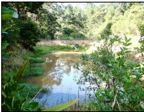
This stormwater management pond is used to control the quantity and quality of stormwater runoff from the Kay Road Balefill which helps to protect the Billy Joe Stream
