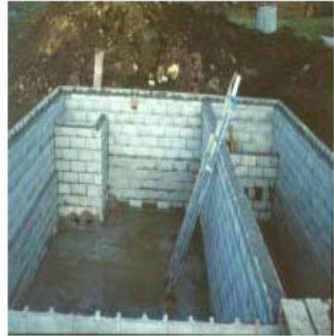
Figure 6: Road Stormwater Sand Filter
