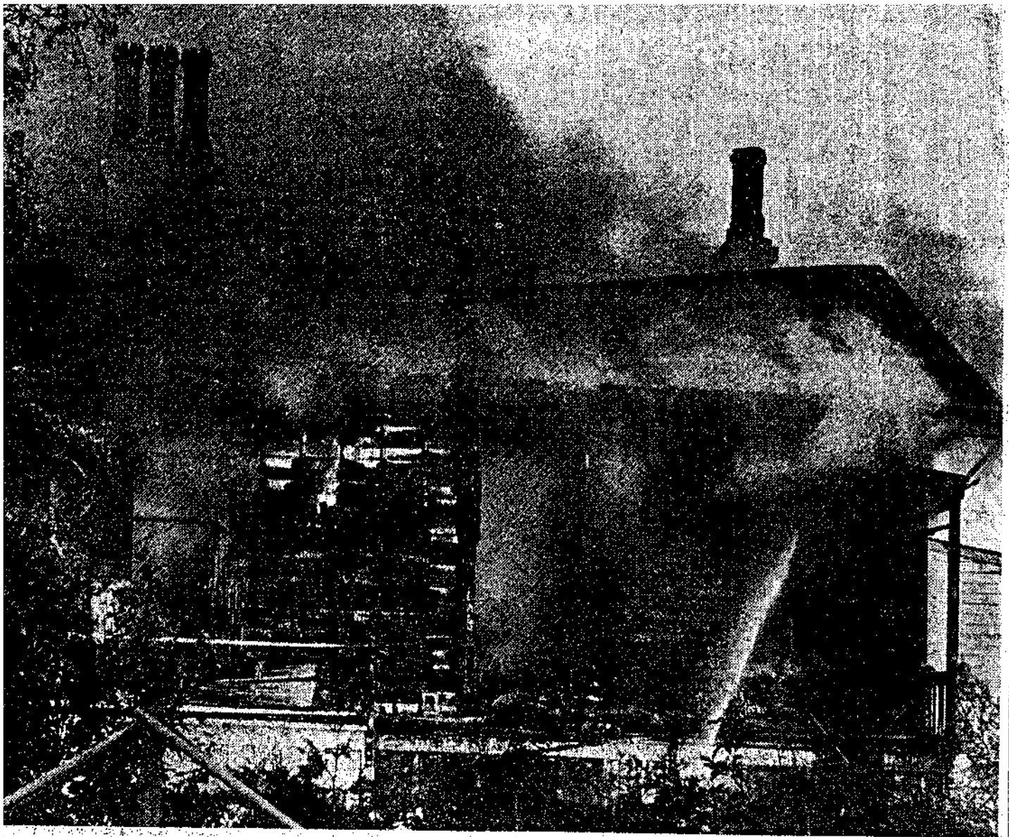
The upper storey of the yoga centre at Henderson during the fire yesterday.
