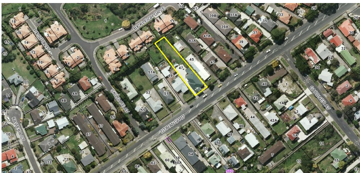
Figure 1: 2008 Aerial photograph indicating the subject site to be subdivided and the existing building
