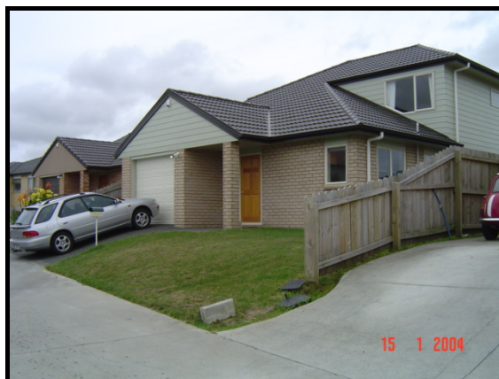
Figure 2: Subsequent Unit: 12 Lucienne Drive
