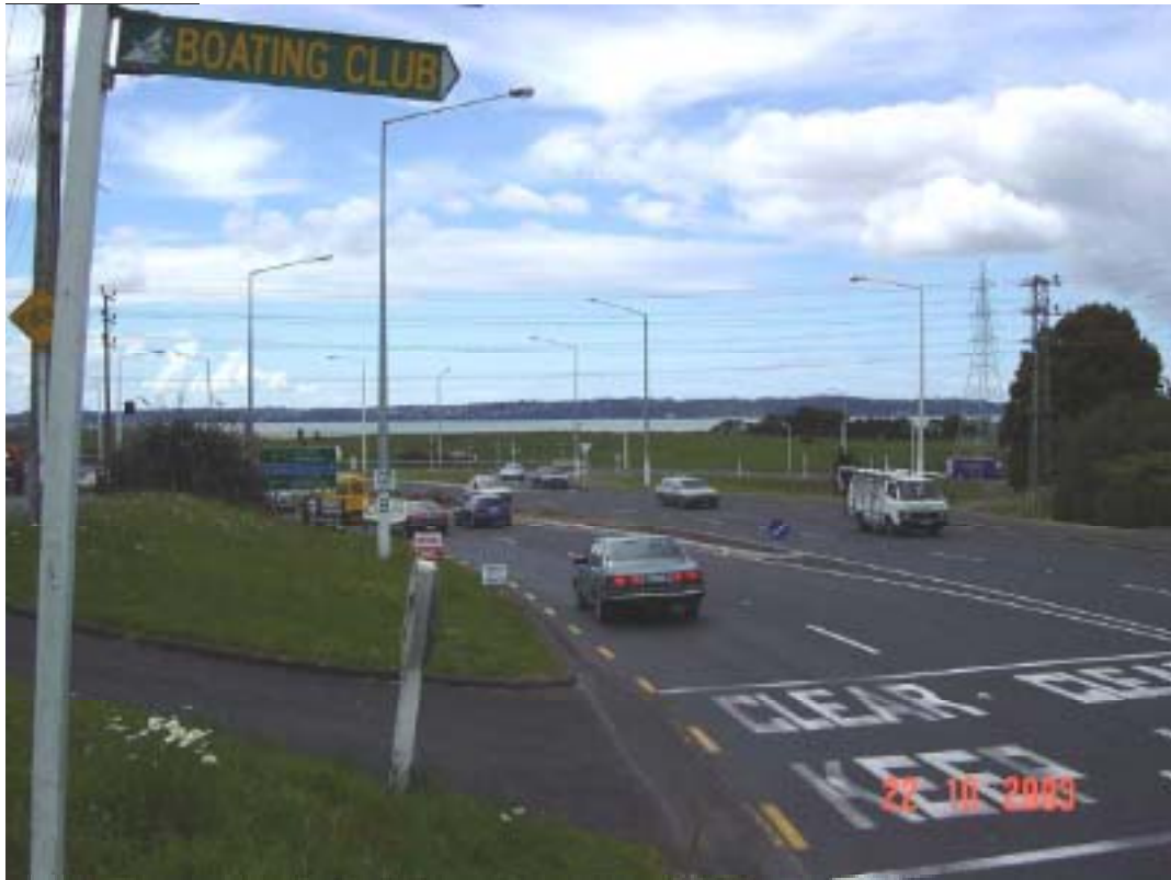
View Adjacent To 356A Te Atatu South Road
