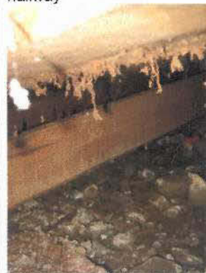
Ground level at back of building in hallway
