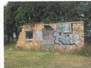
Outhouse west facade
