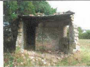
Outhouse north facade
