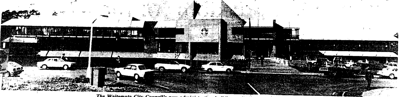
The Waitemata City Council's new administration building at Waipareira Ave, Lincoln.
