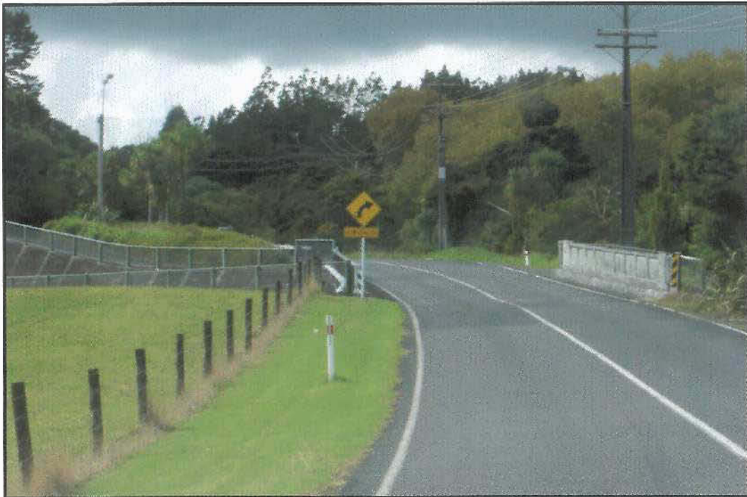
Photograph E: Sign indicating right hand curve when vehicles in fact must make a relatively sharp left turn before turning right
