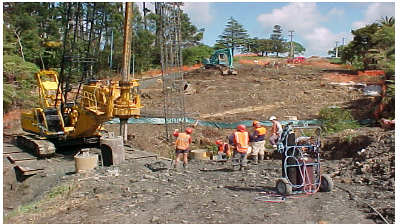
Construction starts September 2004
