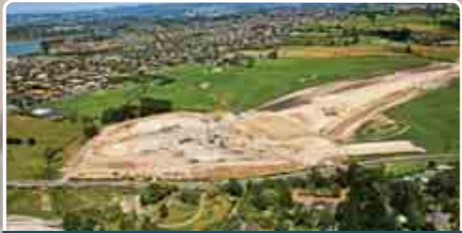
Construction of the roundabouts is underway along Brigham Creek Road
