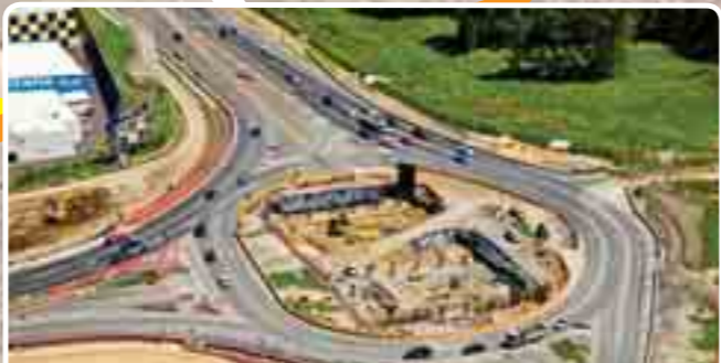
Work continues inside the roundabout at Hobsonville Road
