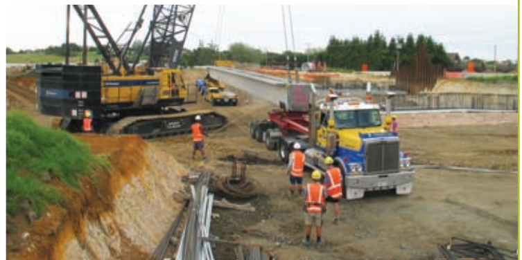
The beams of Trig Road Bridge are lifted into place
