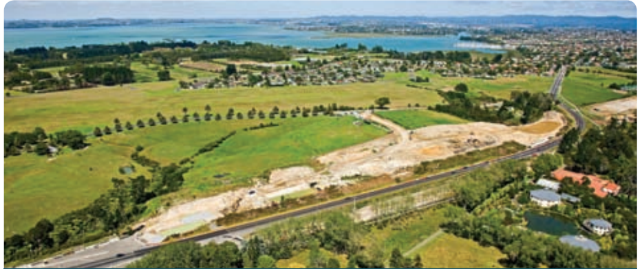
The new Squadron Drive Interchange under construction near Monterey Park
