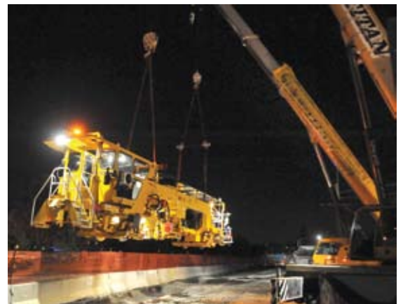
Tamper being craned onto new track
