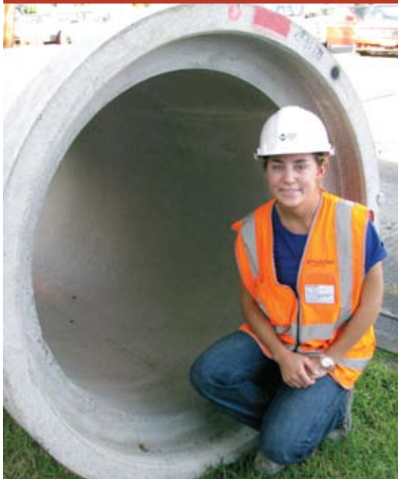
Site engineer Amy Hodgson with one of New Lynn's new 1050mm diameter stormwater pipes
