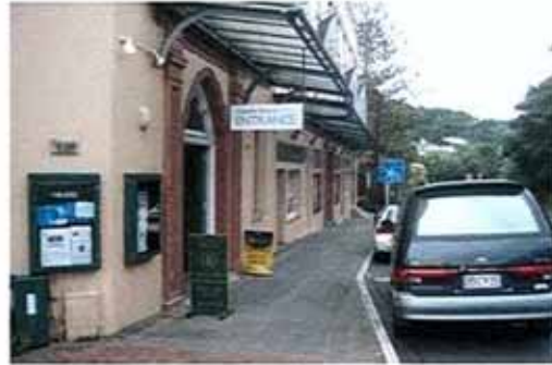
2 Lopdell House street frontage
