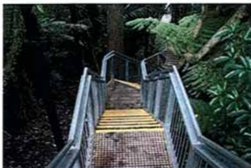
15 Access stair to carparking area at 500 South Titirangi Road
