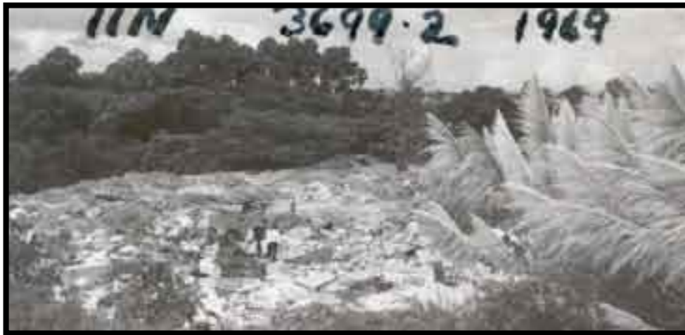
Tip In Old Clay Quarry - From Margan Ave 1969 (J.T Diamond Collection) Waitakere Library and Information Services Photograph Collection
