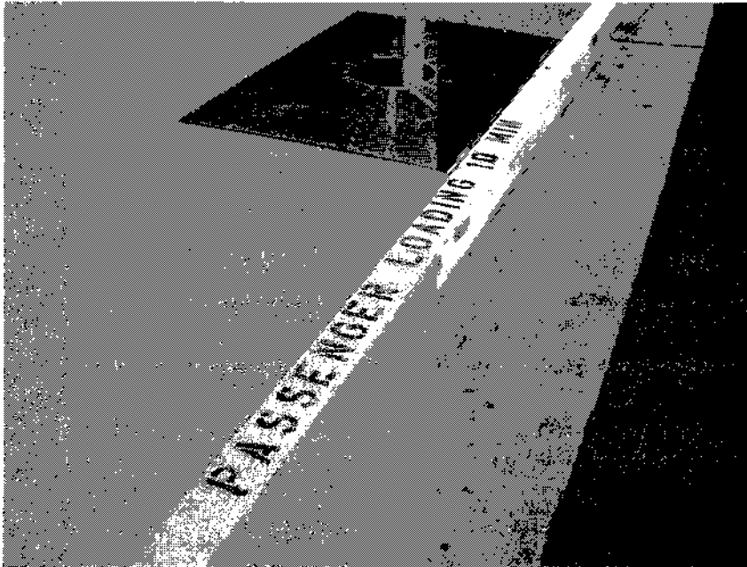
Example of Signage Painted on Kerbs in San Diego California
