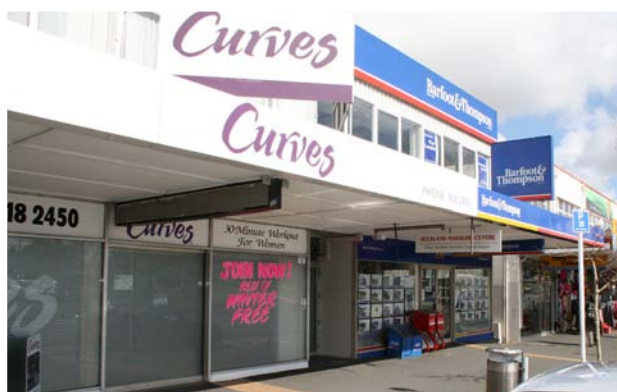
Figure 3.27 Glen Eden Main Street – Limited activation of north facing frontages
