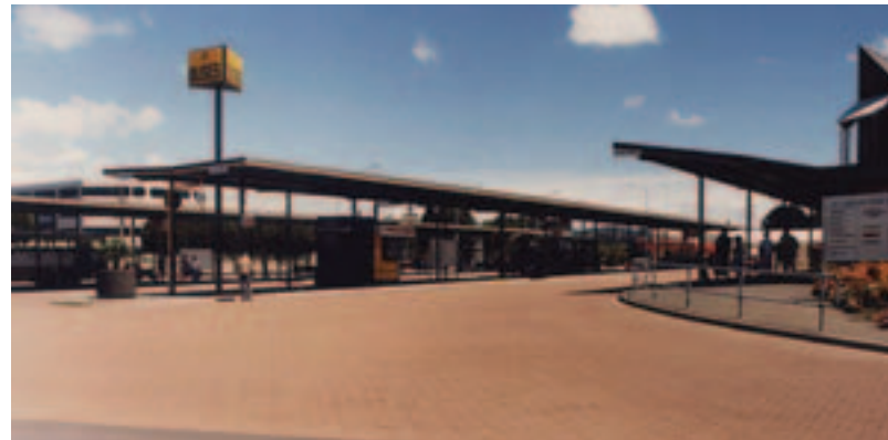
New Lynn's bus interchange is to be re-established to fit with the railway station and town centre.
