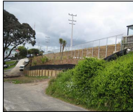
Slip remediation and pedestrian access
