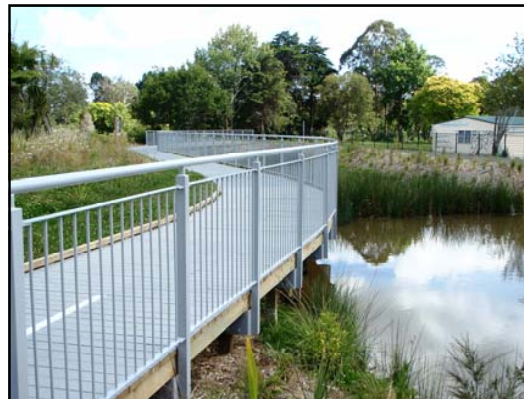
Projects delivered that promote safe walkways/ cycleways for community use
