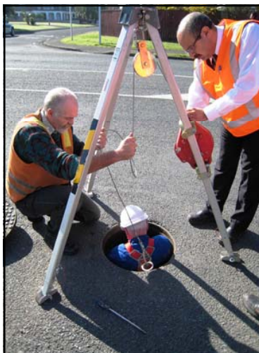
Independent quality control inspections
