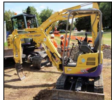
Delivery of projects underground
