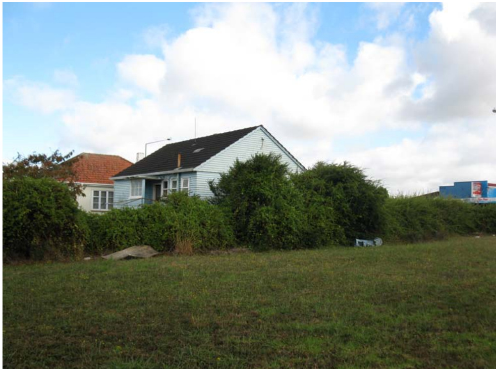
Picture 1: View from 3178 Great North Road, New Lynn towards the existing dwelling at 3180 Great North Road, New Lynn.
