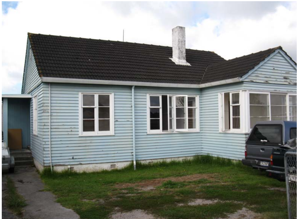
Picture 3: Existing dwelling at 3180 Great North Road, New Lynn.
