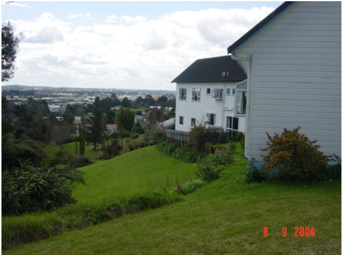
Photograph one - existing rest home located at 19 Denver Avenue, Glen Eden.
