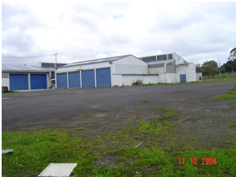
Image 2 - Loading area located at the rear of the main building on subject site
