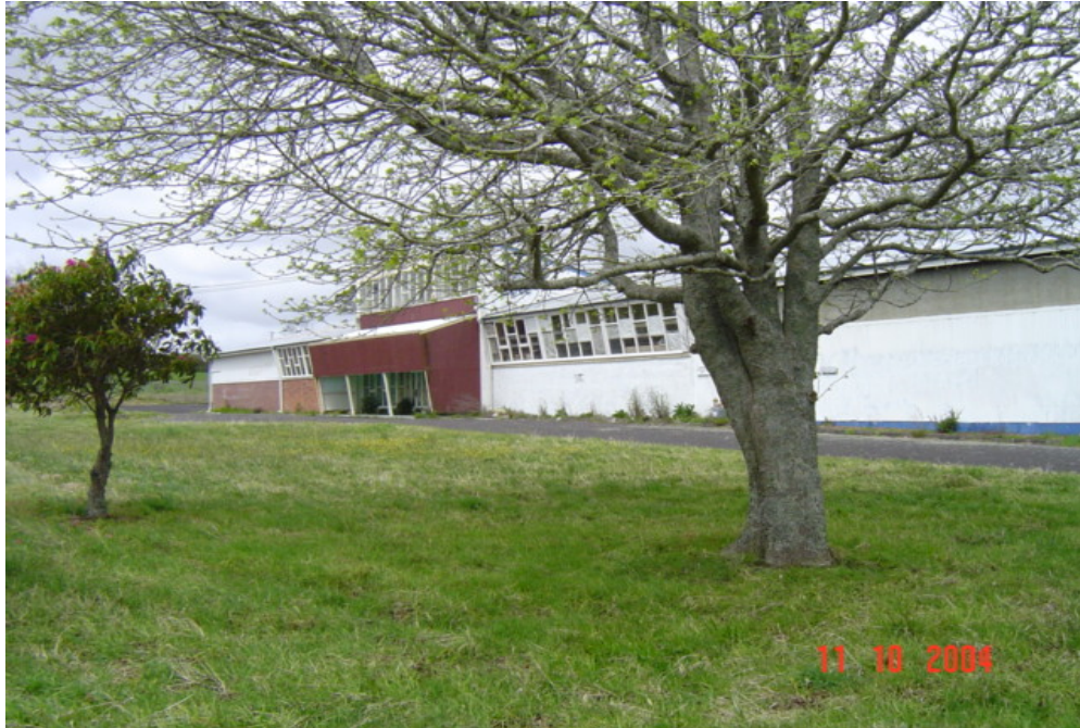
Image one - exterior of main building on subject site
