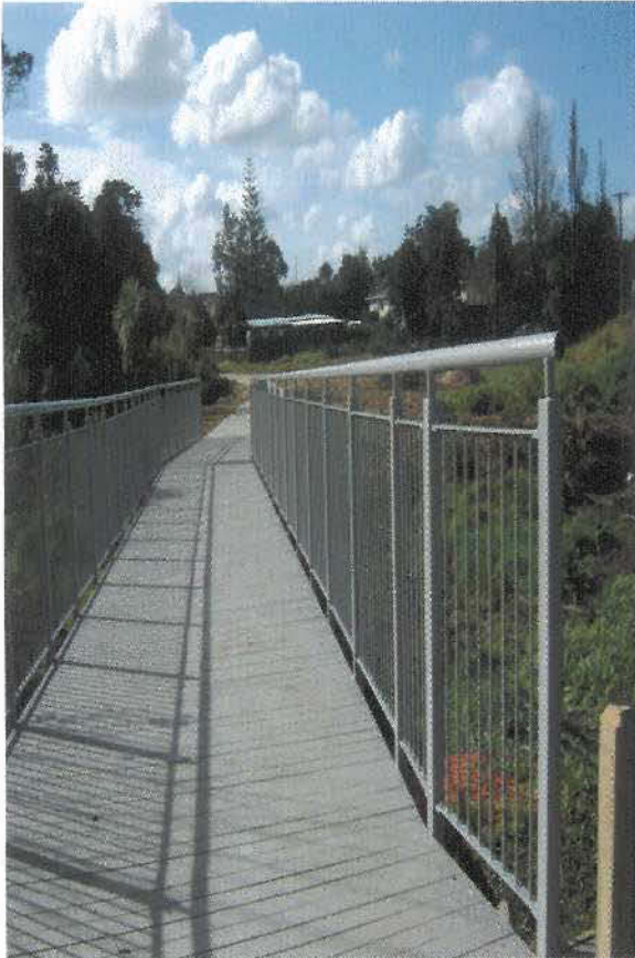
Example of bridge with Parks Standard Handrail – above, and boardwalk below.
