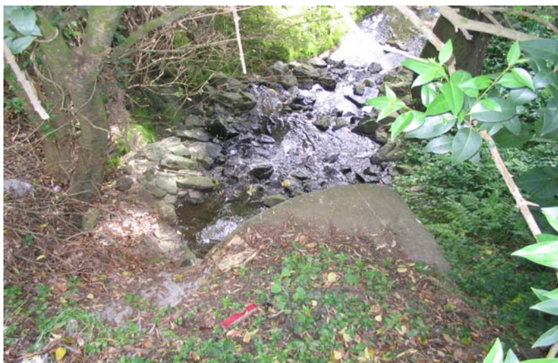
Photograph 2 - Culvert located at Chainage 430.
