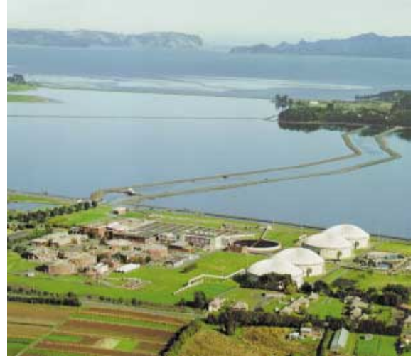
Mangere Wastewater Treatment Plant
